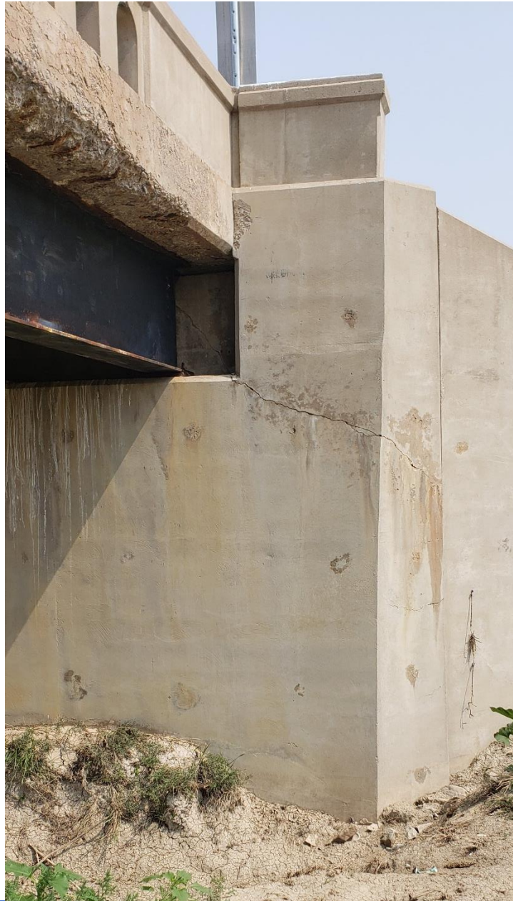
EXISTING BRIDGE ABUTMENT WITH CRACKING STRUCTURE M-21-B FIGURE 2
